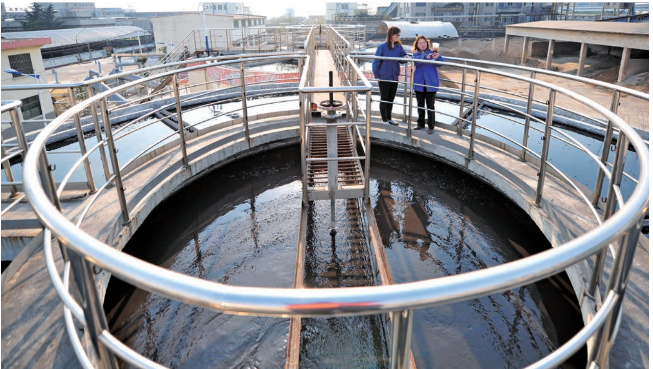
Mine water efficiency sedimentation basin
