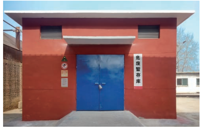
Hazardous waste storage warehouse
