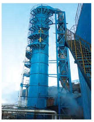
Desulfurization tower of boiler flue gas treatment and transformation project
