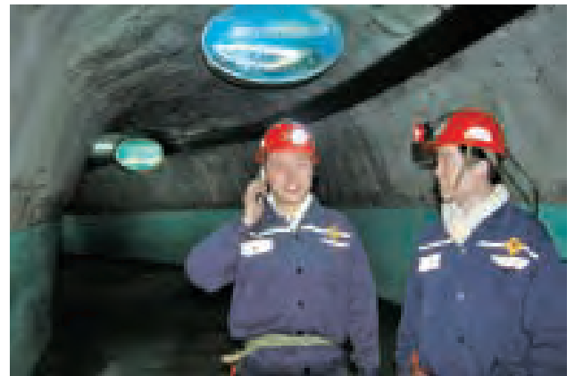
Wireless telecommunication system for mine use
